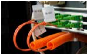
Fiber Optic Cable Markers
